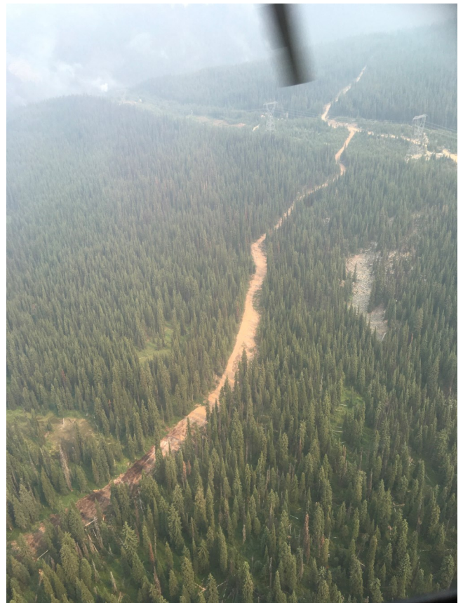
Top: Control line being constructed on Octopus Creek Wildfire (July 31, 2021)
